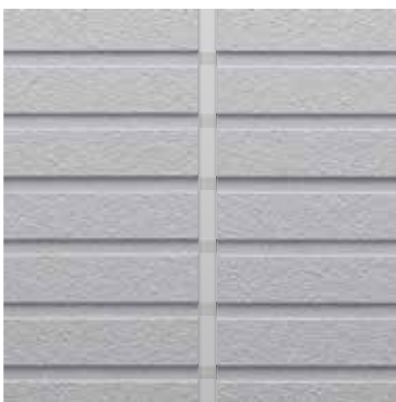
When using caulking
